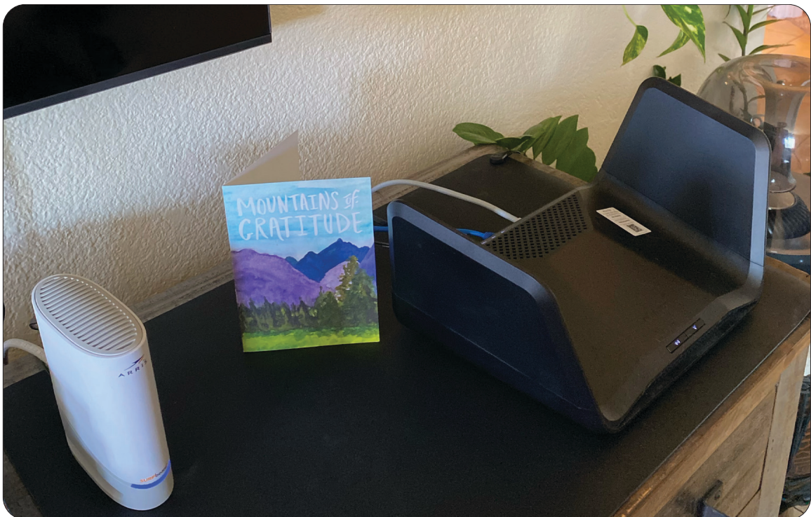
FIG 7. MODEM AND WI-FI ROUTER GROUNDED
